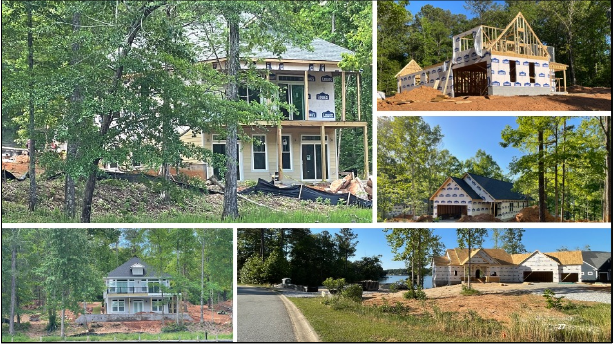
NEW HOMES BEING CONSTRUCTED
