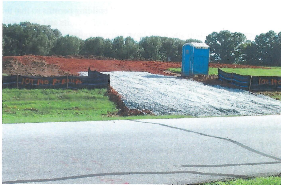
Example of Required Erosion Control using silt fence and rock driveway
